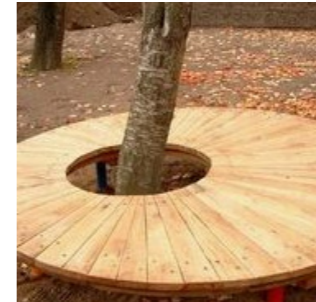
An informal bench wrapped around a tree - tree branches lifted to 2m - laving a gap between tree and bench to allow the trunk to expand as the tree grows. The tree bench will be wider on one side than the other, making it playful and a space for erpose. The tree bench is set back from the main path to give a sense of privacy and enclosure.
