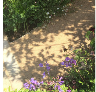
The path is made up of 15 circles connected with curvaceous lines, making visual reference to #Challenges15. The path takes the visitor of a journey through the gardens linking the seating spaces and creating a meditative route to walk. Made of a self binding gravel, CEDAC and edged with CEDAREGDE 150mm metal edging, edging to rise 50mm above final path level.
